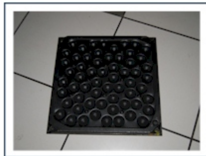
2. BOTTOM OF FLOOR PANEL
