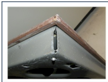
4. CORNER OF FLOOR PANEL
